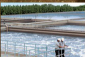
WATER TREATMENT SYSTEMS
